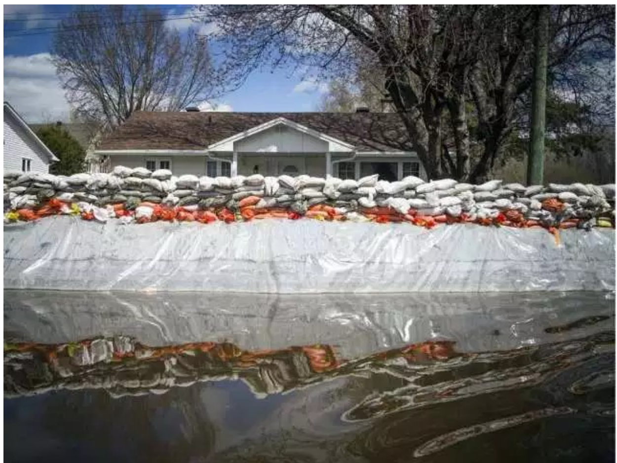
A wall of sandbags protects a home on Rue de Versailles. Ashley Fraser / Postmedia
