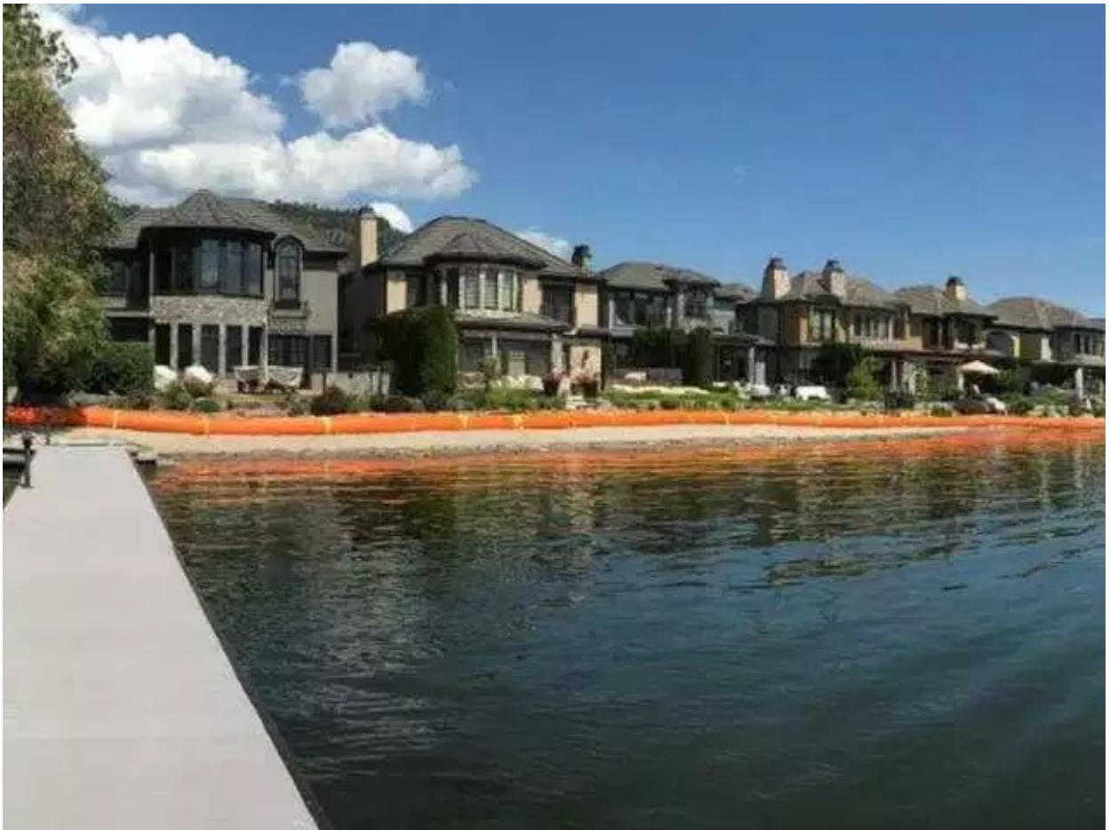
A Tiger Dam tube is used to protect homes from flooding in Kelowna, BC, in 2018. jpg
