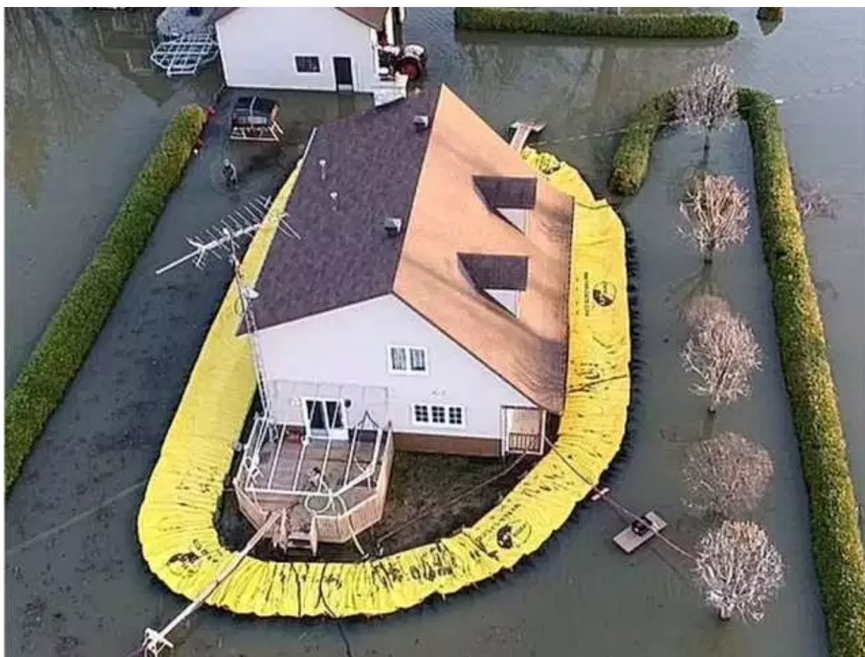
The Water-Gate, a portable flood-prevention device, in used during 2019 flooding in Rigaud Quebec. jpg
