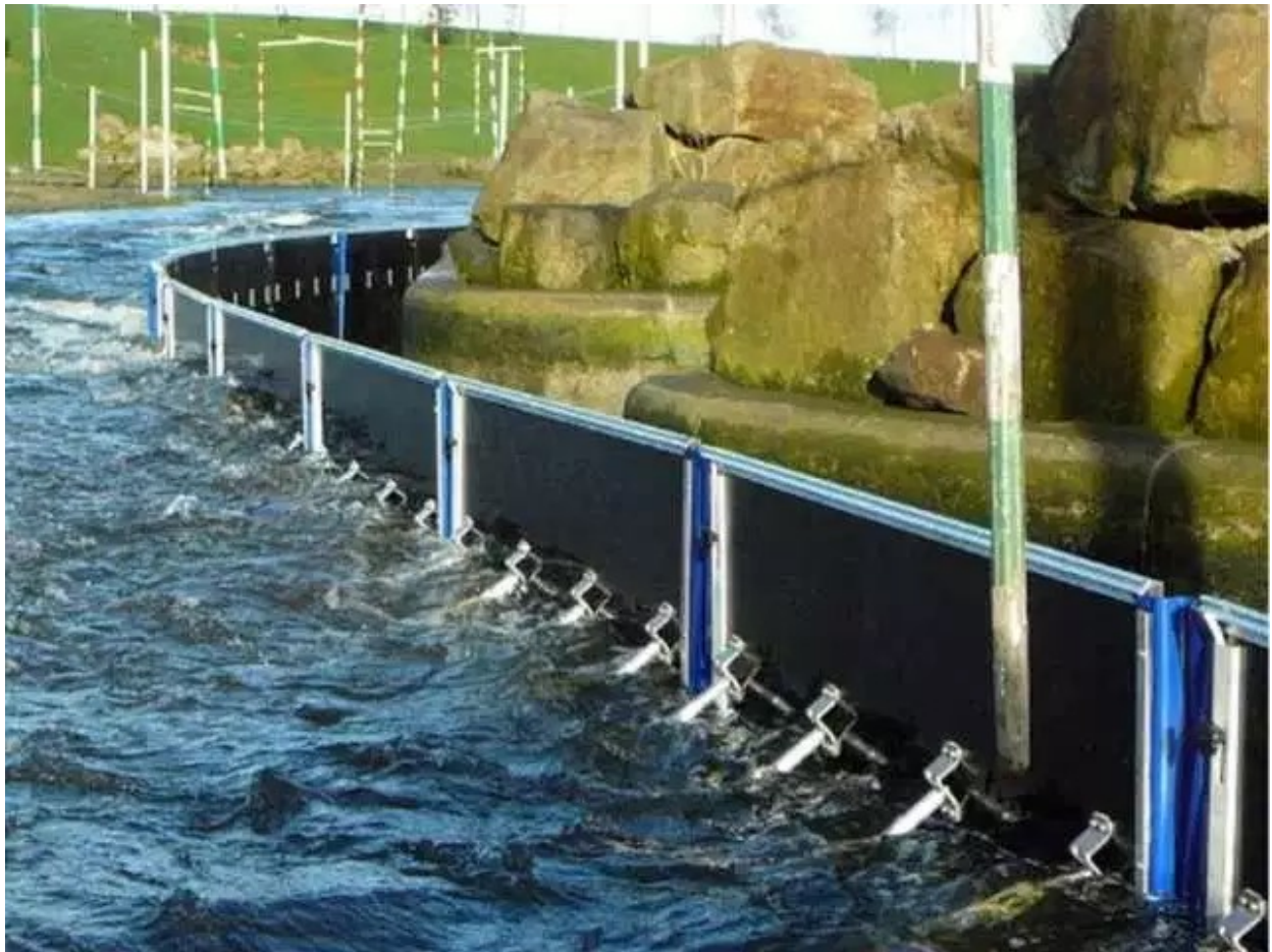
The WaterFence is a portable flood barrier developed in Norway. jpg
