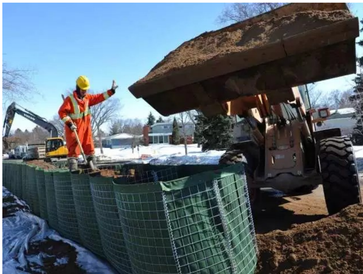
City of Regina crews fill large collapsible lined frames known as HESCO barriers for flood protection in April, 2013. ROY ANTAL / THE CANADIAN PRESS
